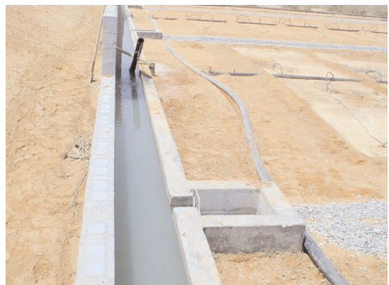
Treatment of oil process water and biosaline agriculture pilot project at Nimr, Oman. Reed bed irrigated with oil process water (above). Treated effluent from the reed bed (below)
