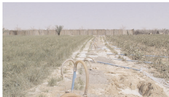
Dewatering for installation of drainage system
